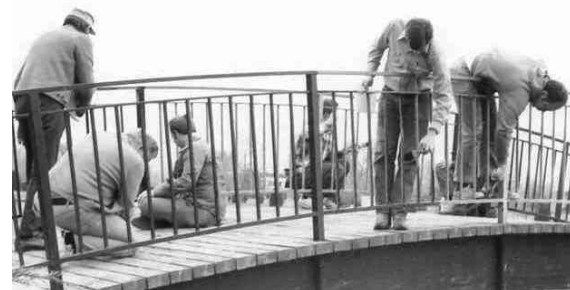
Painting Greenbelt Bridge—1979
